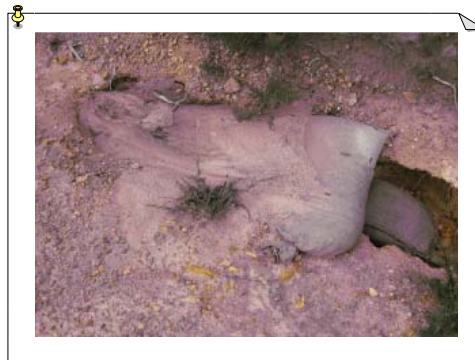
“hard working sand bag” : A couple of sand bags in an eroding road drain—one rain event and it filled to the top with sediment! Submitted by Matthew Hulse, Braidwood
