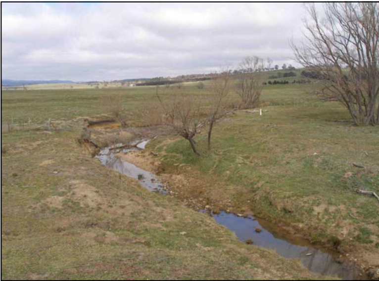
Turallo Creek adjacent to Kings Hwy near Bungendore – before & after a deluge.
